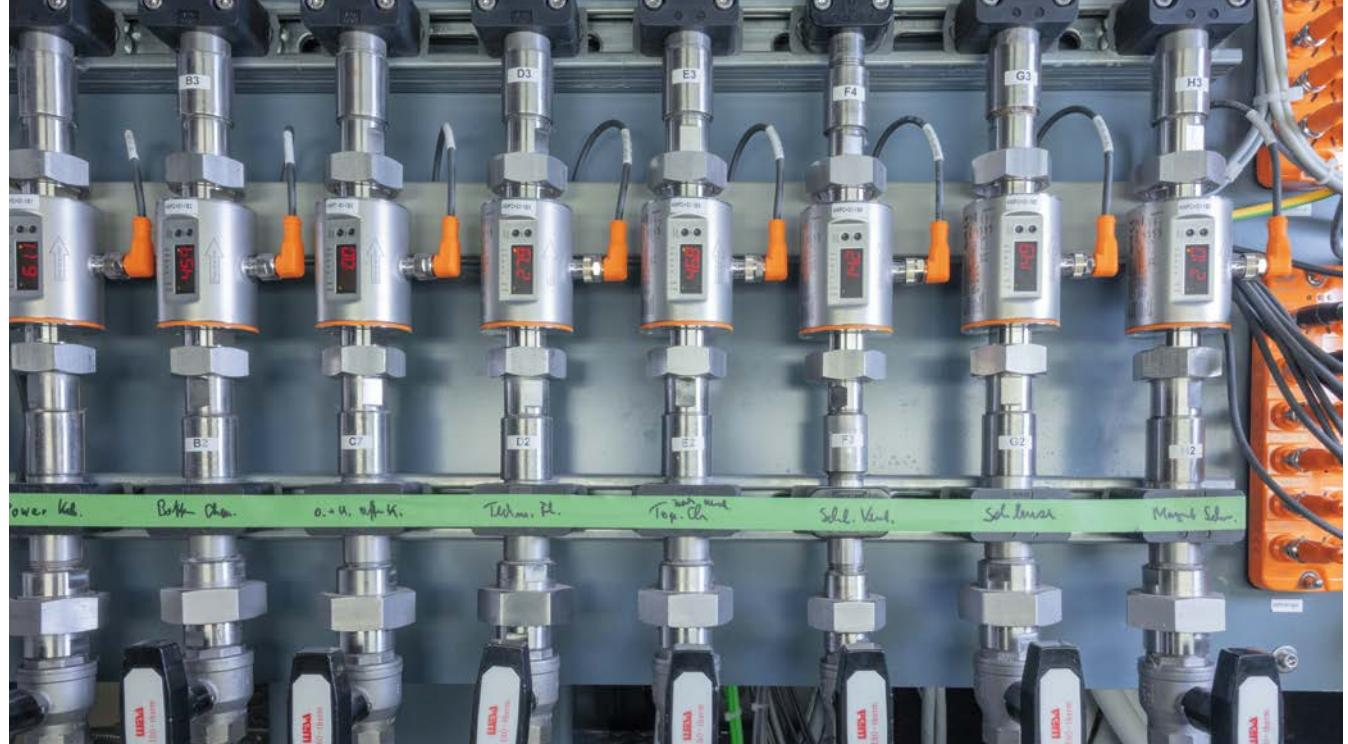
*Flow sensors monitor the cooling circuit of the Czochralski system.*
