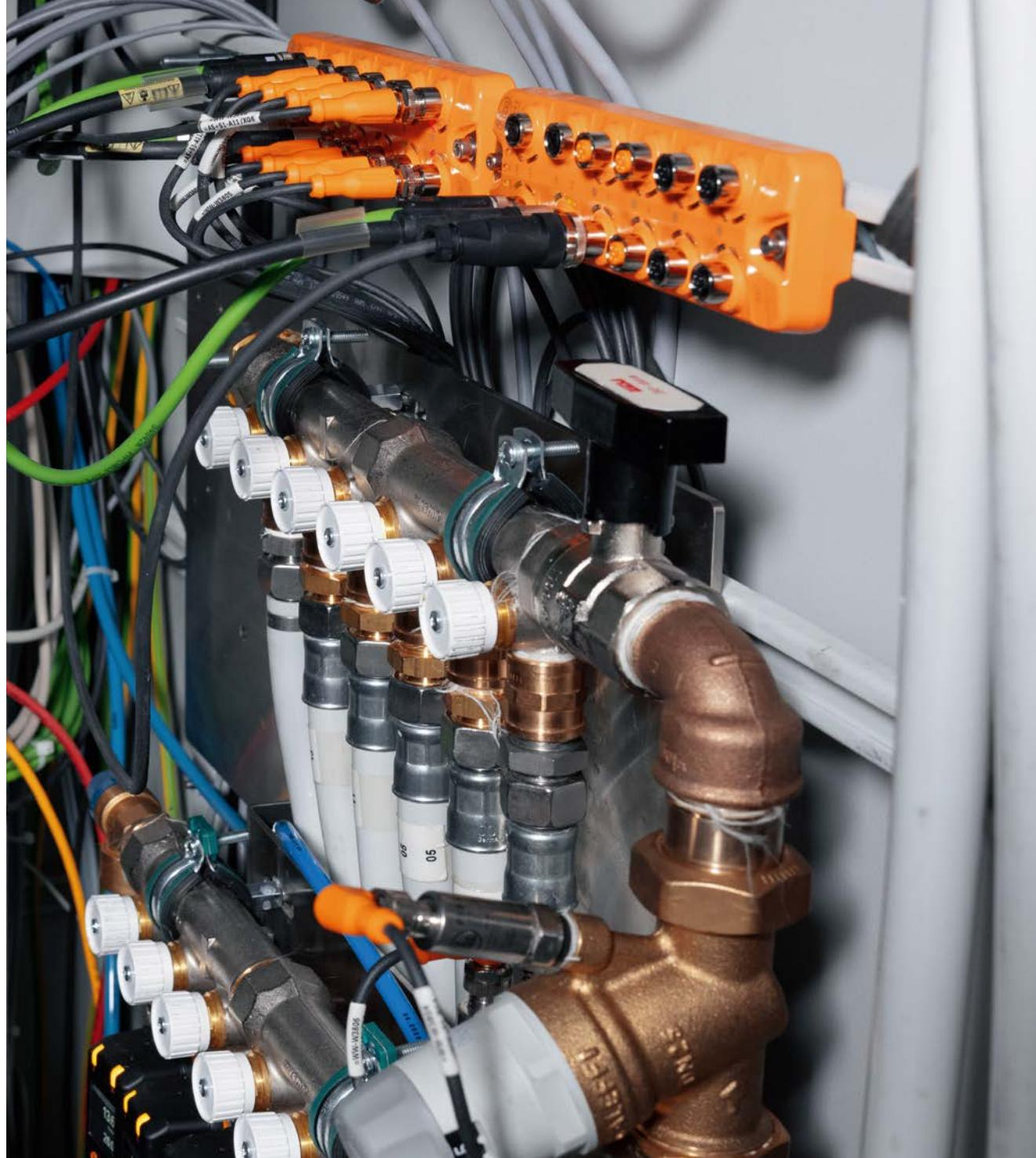
*The IO-Link master (top) collects and forwards data from the pressure sensor (centre, front) and the flow sensor (lower left).*
