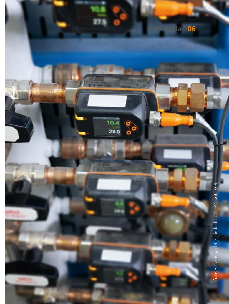
*Easy to read: flow sensors on a diffusion bonding system.*
