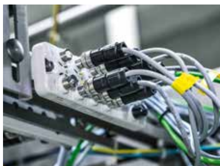
Decentralised IO-Link modules bundle the sensor signals while enabling a detailed insight into the digital sensor from the IT side, which allows for extensive diagnosis.
