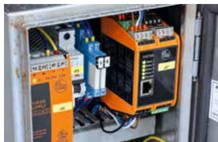
The VSE100 evaluation unit evaluates the signals from up to four vibration sensors.
