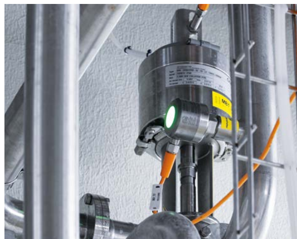
For particularly process-critical locations: self-monitoring temperature sensor TCC with visual status display.
