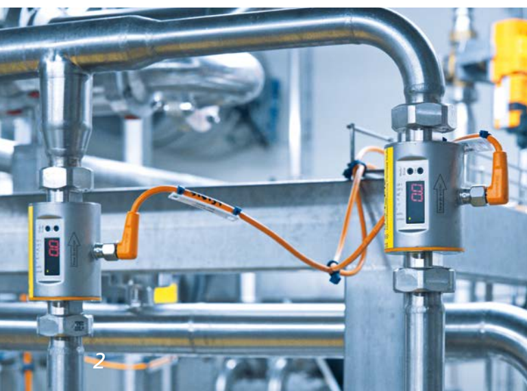
Magnetic inductive flow sensors in the permeate stage of the reverse osmosis system monitor and control the concentration of the whey.
