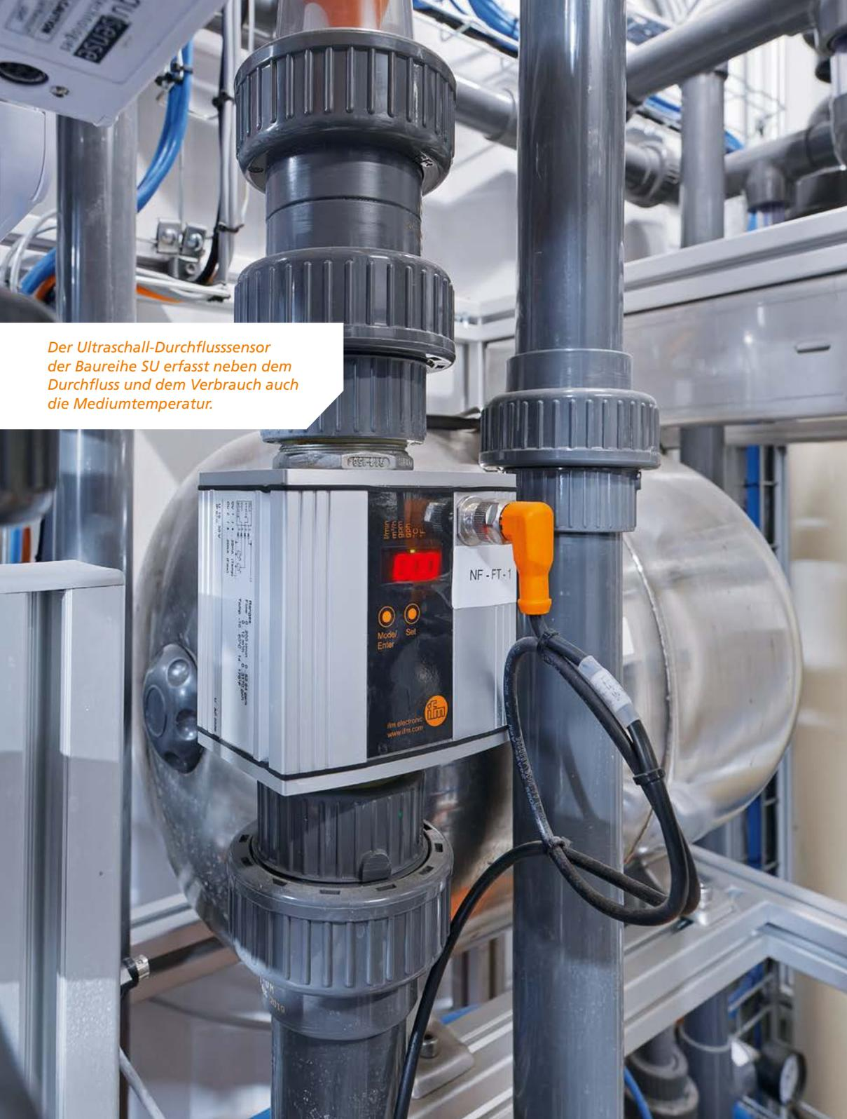
A vertical grey pipe assembly with a white rectangular sensor box mounted on it. The sensor box has a red LED display showing '0.00', two orange buttons labeled 'Mode/Enter' and 'Set', and a label 'NF-FT-1'. A black cable is connected to the side of the box. The background shows industrial equipment and blue hoses.
