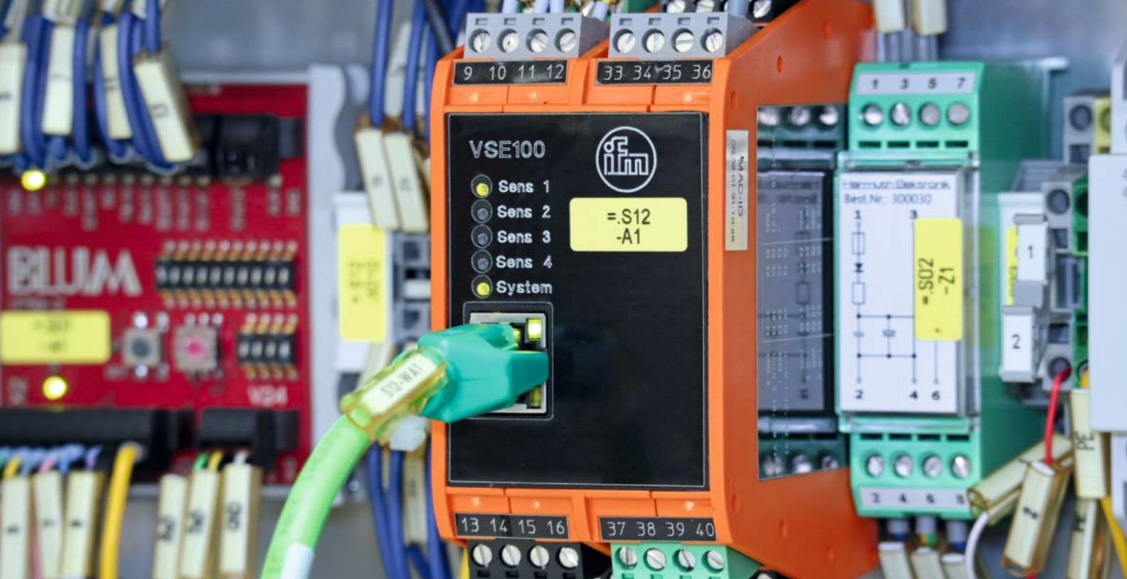
Processes the vibration signals from up to four sensors: the VSE100 evaluation unit.
