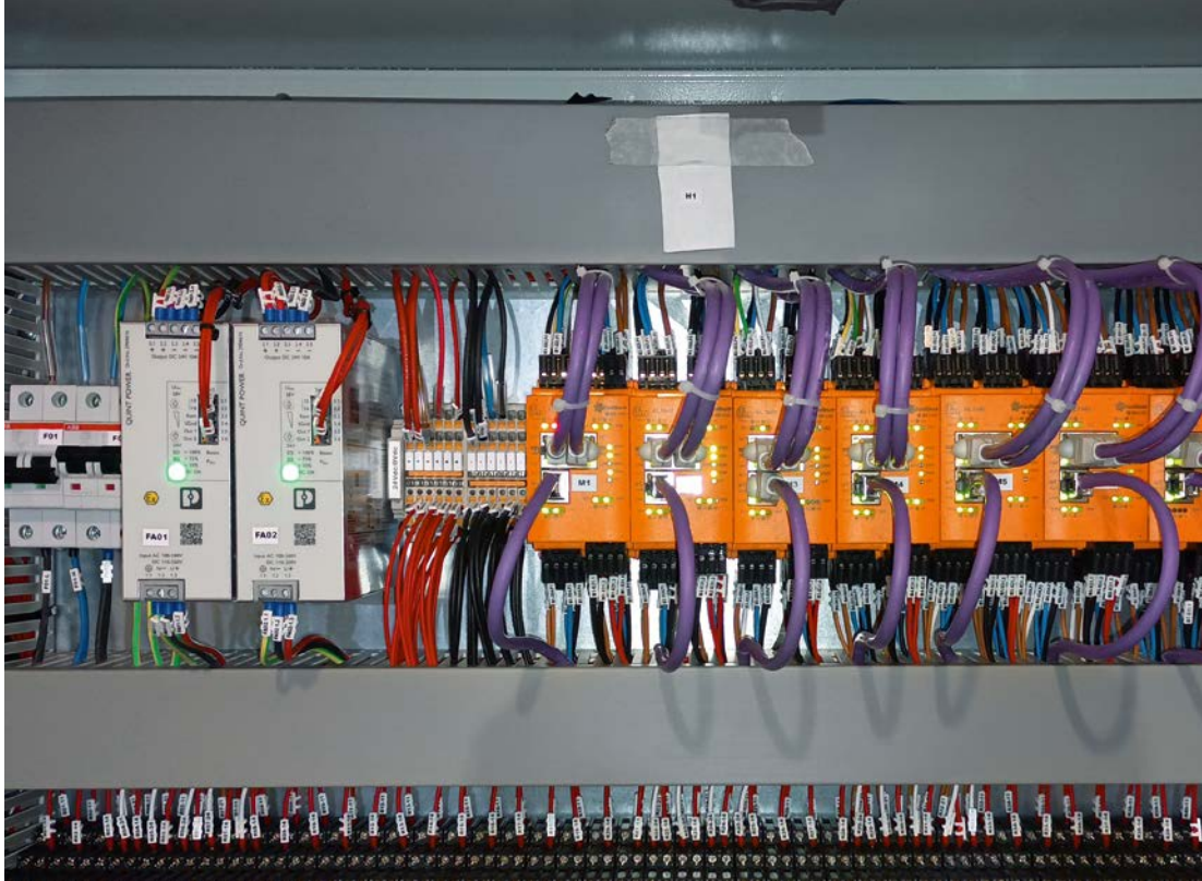
IO-Link masters and evaluation units for vibration sensors collect the data and transmit it in consolidated form to the IT level.
