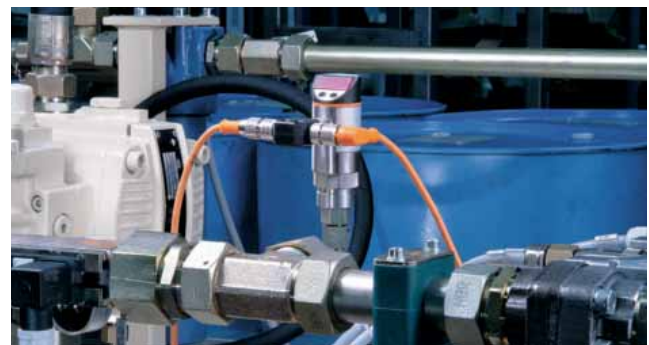
Differential pressure measurement in filter monitoring.
