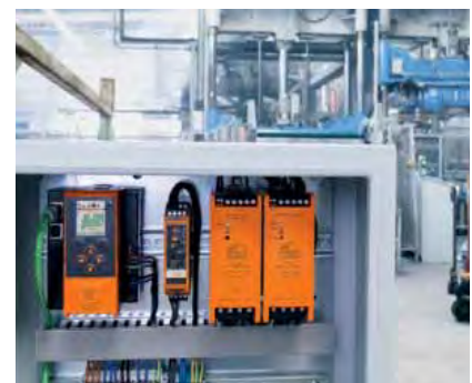
Gateways allow connection of AS-i to different fieldbuses.
