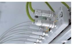
Subsequently, the wort from the brewhouse can be matured in the fermentation and storage cellar to finish the beer and is reliably secured by self-monitoring temperature sensors without the risk of temperature deviation. These sensors are connected directly in the field via IO-Link masters, which saved Doemens a considerable amount of wiring. Even cleaning processes are no obstacle to using the masters directly on the plant.
