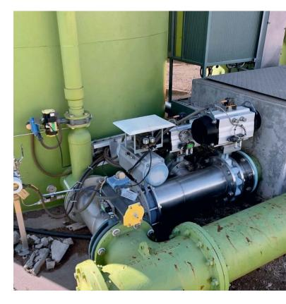
the time for implementation is reduced thanks to the master connection, because the parameters are saved on the master and are automatically written to the new device after the sensor is replaced. For Lower Murray Water that means seamless and reliable monitoring of the backflushing process is guaranteed at all times.
