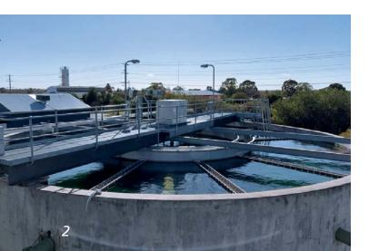
The untreated water passes through several stations as it is treated to become drinking water, including filtration. During this step in the process, tiny suspended particles that have not already been removed from the water by flocculation, precipitation and sedimentation are filtered out. Since the filters become increasingly blocked as particles settle on them, they must be cleaned regularly by means of backflushing. This is the only way to retain functionality and the flow of water.
