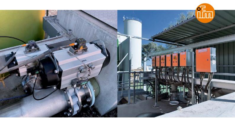
The MVQ101 ensures a reliable separation between drinking water and industrial water. The sensor detects even the smallest opening of as little as 0.1 degrees.
