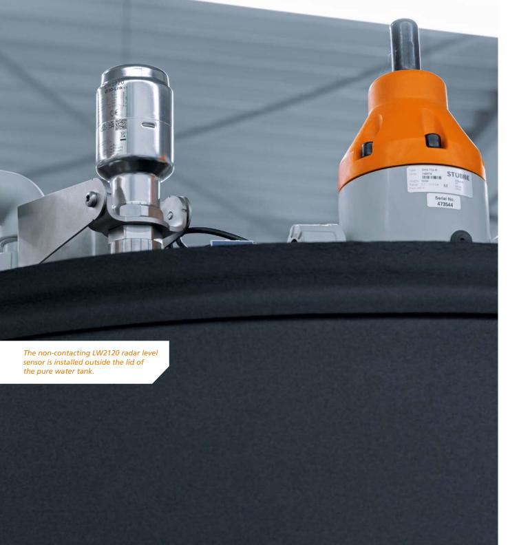
Standard M12 connection technology ensures error-free installation within minutes, while IO-Link adds the convenience of remote parameter setting and reading. The intelligent algorithm in the unit makes parameter setting via IO-Link seem like child's play: After setting the reference height once, the sensor immediately provides the exact level via IO-Link.
