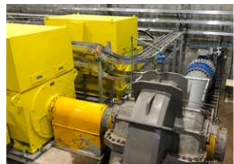
North Otago Irrigation pump station, employs ifm IO-Link condition monitoring systems. This state of the art pump station transfers 2 m 3 /s
