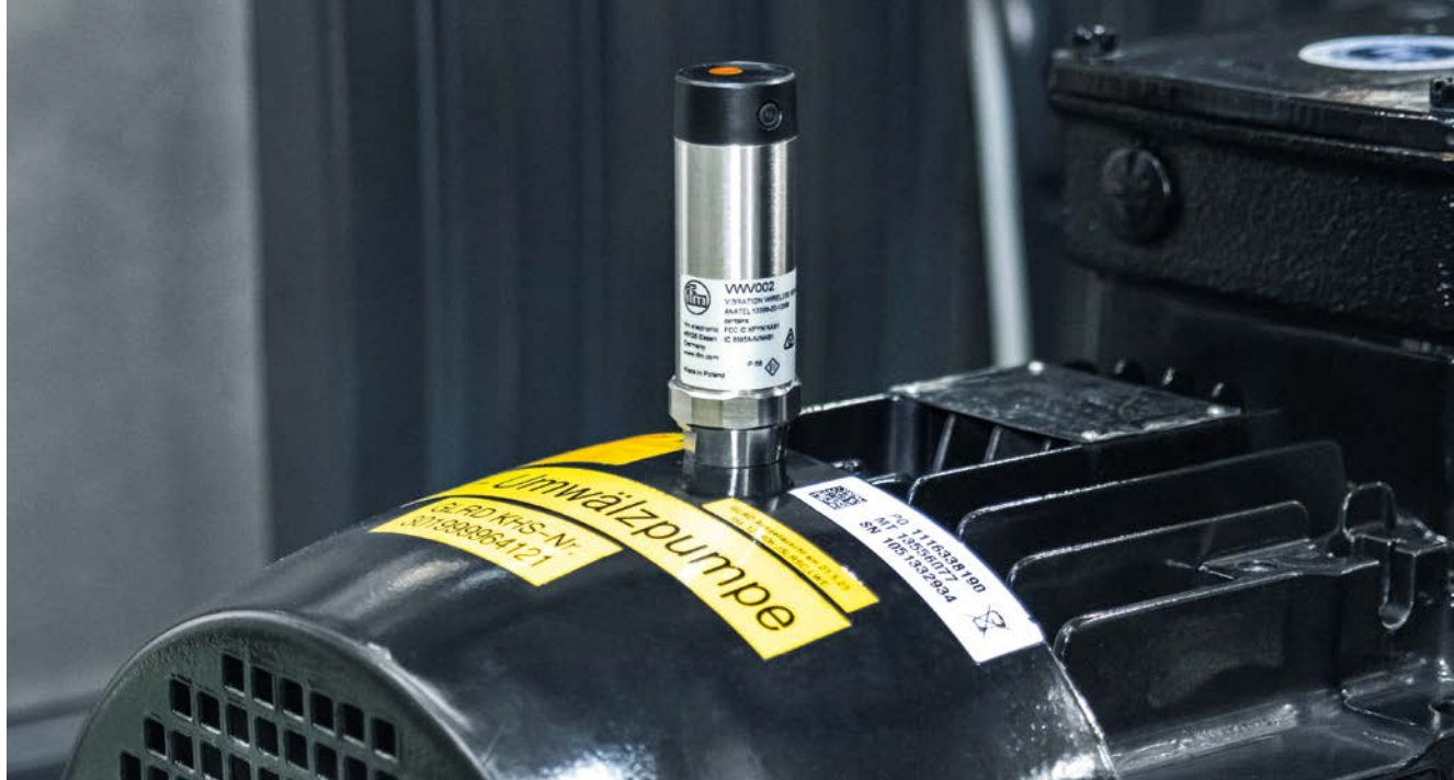
A wireless vibration sensor on the circulating pump for reliable, intermittent monitoring of the total vibration in accordance with DIN ISO 10816.
