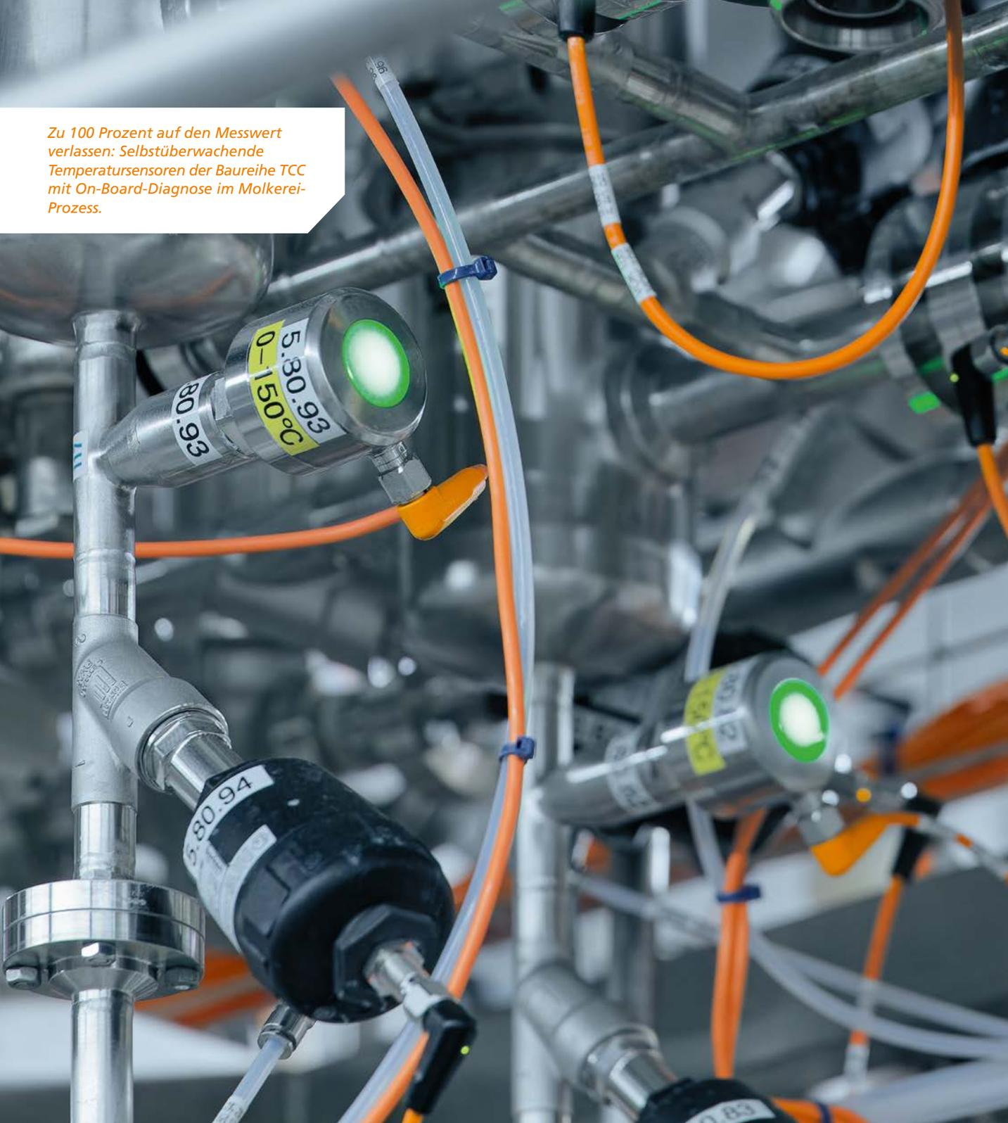
The image shows a close-up of industrial machinery, likely a milk processing plant. Several temperature sensors (TCC) are mounted on stainless steel pipes. The sensors are cylindrical with a green LED light on top. One sensor in the foreground has a yellow label that reads "5.80.93" and "0-150°C". Another sensor below it has a black label with "5.80.94". Orange cables are connected to the sensors. The background is a blurred view of the complex industrial structure.
