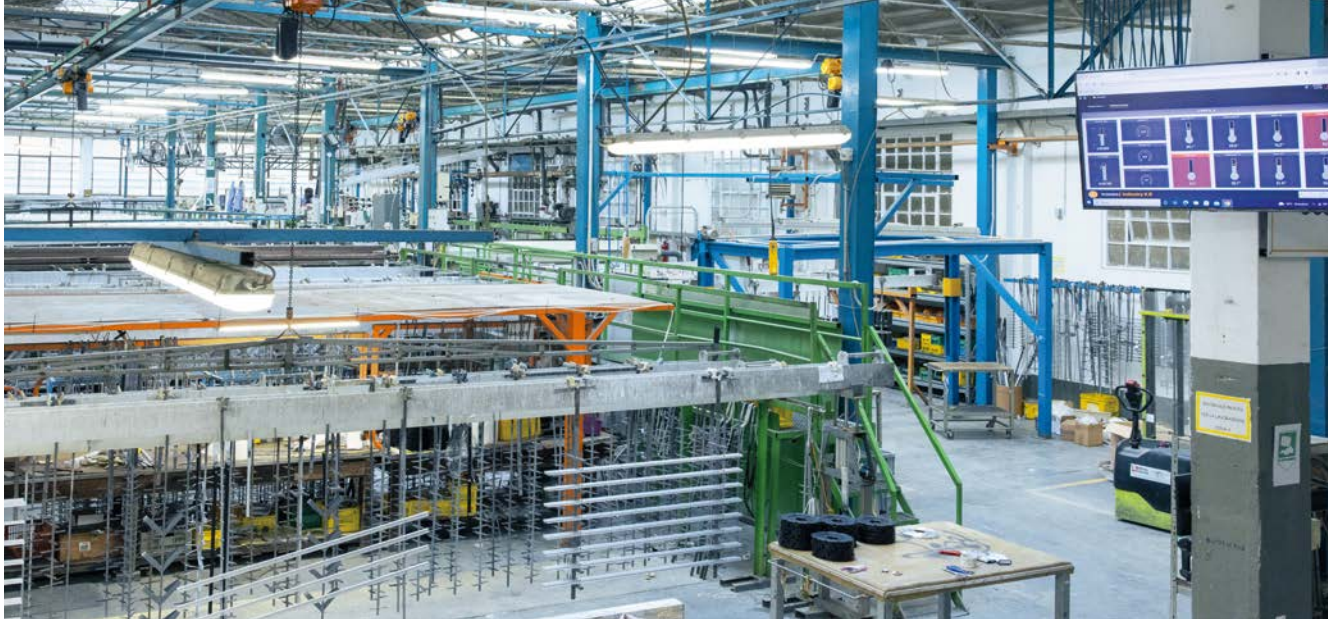
The moneo dashboard with the main process data is highly visible in the workshop. The response time is much shorter when intervention is needed.
