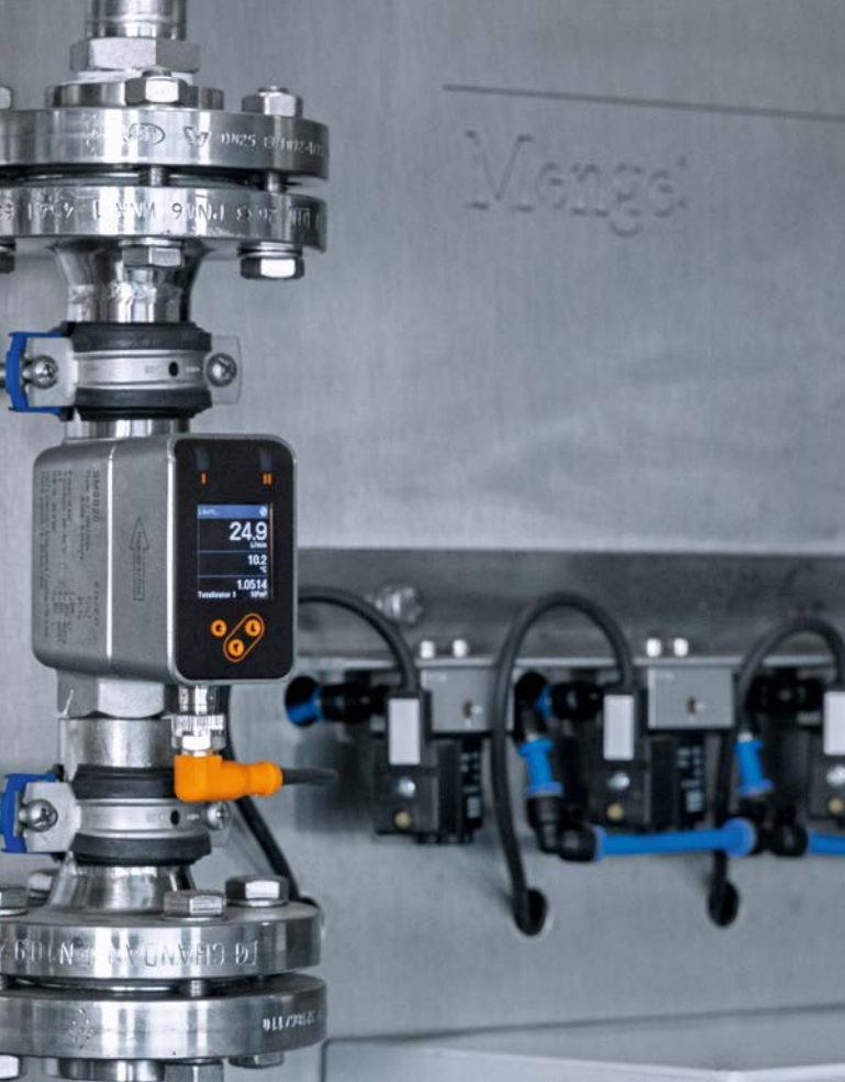
Various flow sensors help with the dosing of the flocculant.
