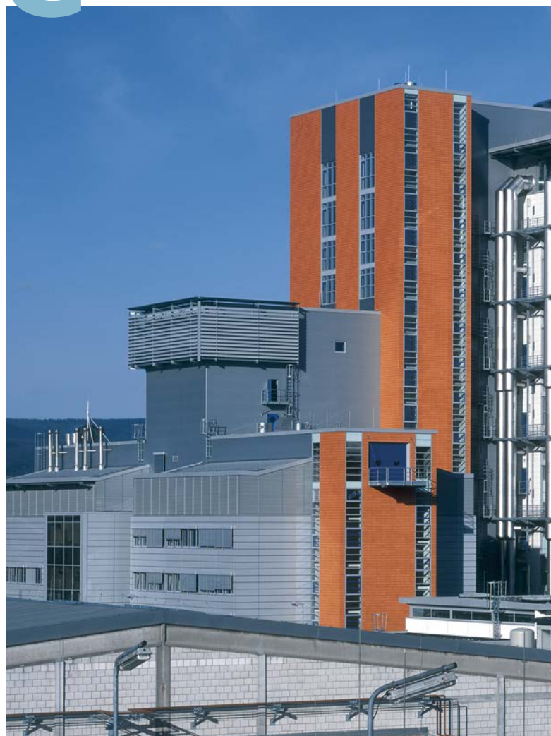
The pharmaceutical company Boehringer Ingelheim relies on vibration diagnostics from ifm for condition-based maintenance in its cleanroom ventilation systems.
