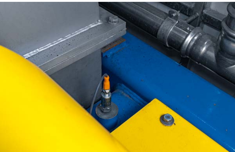
A vibration sensor ensures that no critical vibrations occur.
