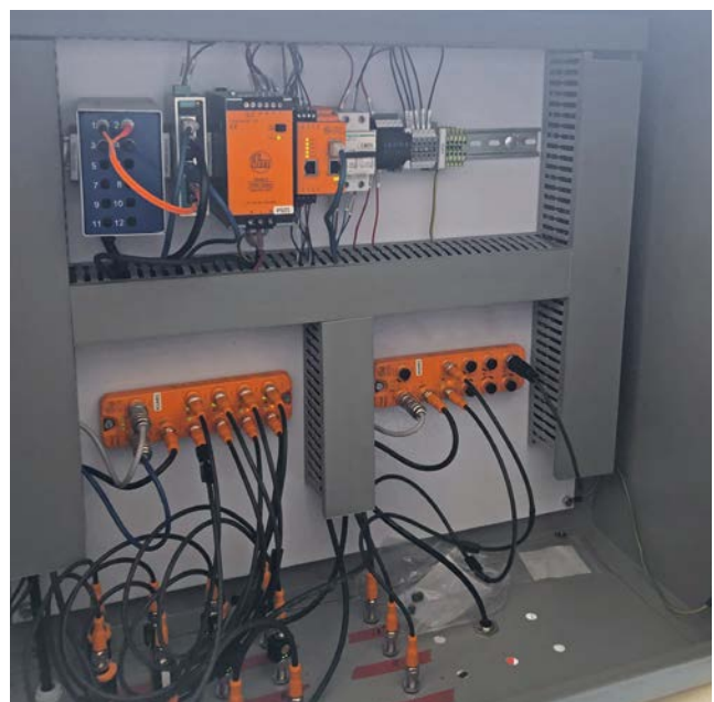
With IO-Link, fewer cables and less space are required. Midvaal Water was able to reduce installation time by 80 percent.
