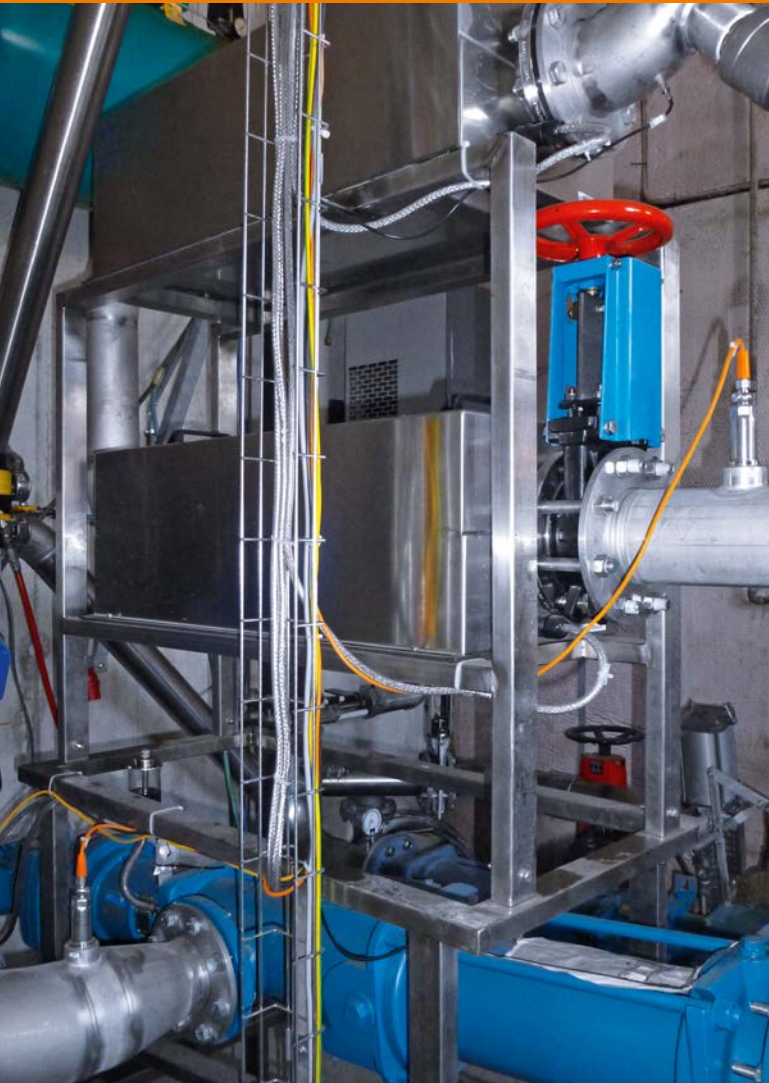
In the ultrasonic disintegration plant, biomass is processed for maximum energy yield.
