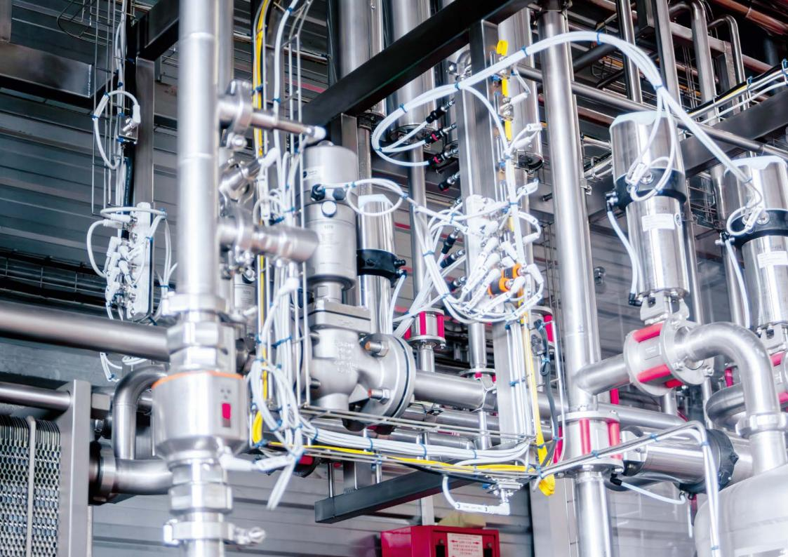
AS-i meets IO-Link: The two digital communication technologies can be ideally networked with each other, harnessing the benefits of both. Here for example, flow, pressure and temperature are transmitted to AS-i via IO-Link.
