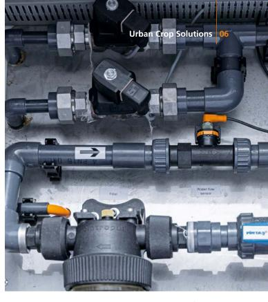
Fill level, temperature, and flow rate – three factors that determine the quality of the plants – are monitored by ifm sensors.
