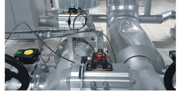
Veltins already has around 40 MVQs in its heating and cooling systems. Data is transmitted either via digital IO-Link communication, or analogue.
