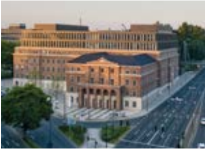
ifm Global headquarters in Essen, Germany
